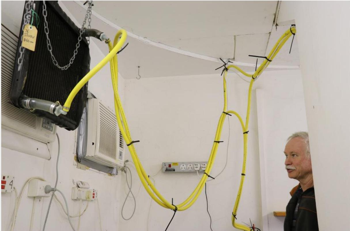
**Mike Hill, electronics technician, with the car radiator he installed to cool the spectrometer at the BiSON station in Narrabri, NSW, Australia. Photo: Tracy Sorensen.**
